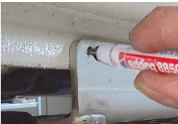
Figure 9: Marking the Holes
